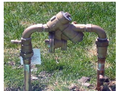
A typical unprotected backflow is easy to take. A covered one is more secure.
